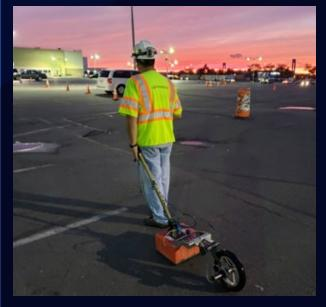
Locating underground utilities using ground penetrating radar
