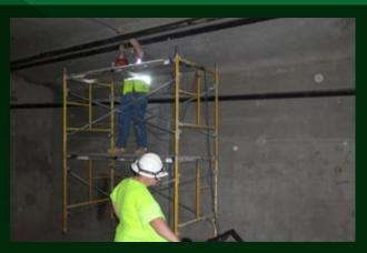
Acoustic testing of external tendon for grout defects, Sarasota, FL
